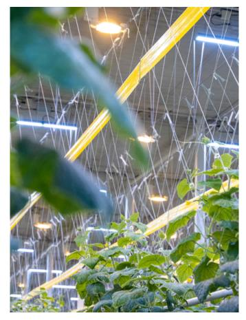
Pictured: Although a full LED retrofit is ideal for optimizing spectrum control, a hybrid system introduces enough LEDs to induce the desired spectrum to enhance plant growth while retaining HPS fixtures.
