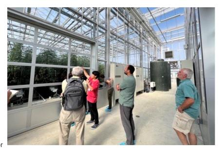
the side walls and state-of-the-art ETFE (ethylene tetrafluoroethylene) plastic film for the roof, which is lighter and more transparent than glass, hail-proof and requires less steel framing to support it. It also has supplemental LED lighting, air circulation fans with a fogging system and a smart shade screen. The goal was to mimic the most advanced greenhouse operations today. They can grow tomatoes, cucumbers, peppers and more in there.
